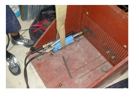
Figure 2 Applying of prestressing force using hydraulic jack in progress
