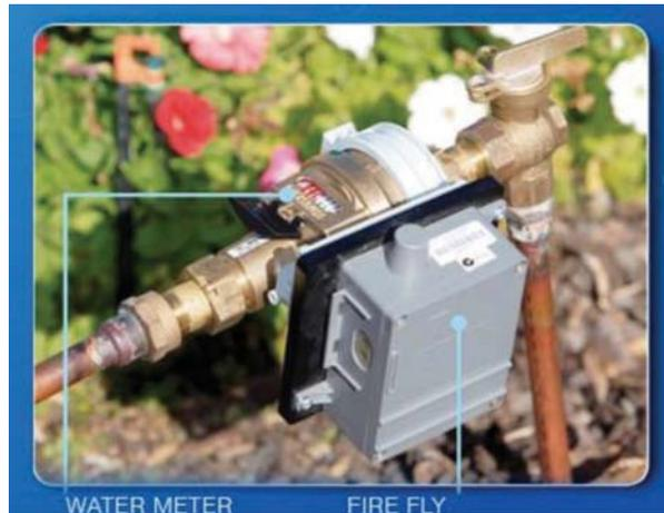
Figure 1. FIREFLY® and Water Meter installation at residential property.
