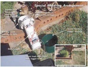
**Figure 5** Smart water meter arrangement on site (Loh and Coghlan, 2003)
