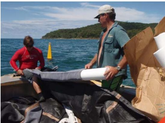
Figure 16: Final assembly and deployment of algae curtain
