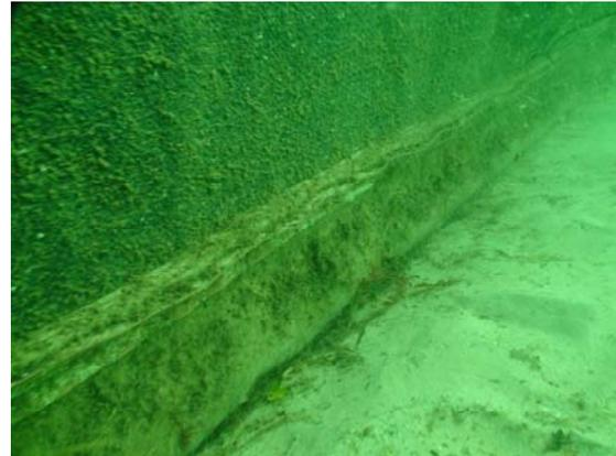
Figure 17: Seabed based algae curtain resting on seafloor
